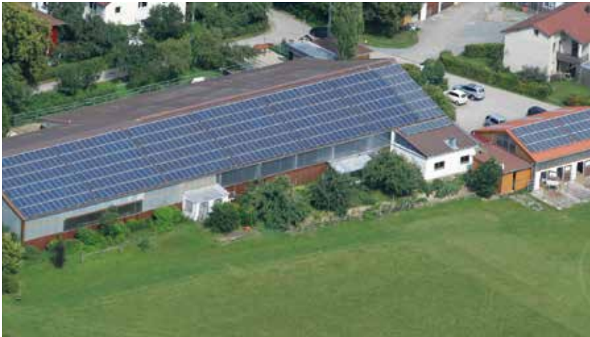
Gäufelden-Nebbringen - Germany System: 31,85 kW | SpeedRail
